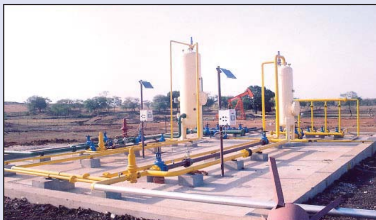
CBM Gas / Water Separation Facilities of RIL
