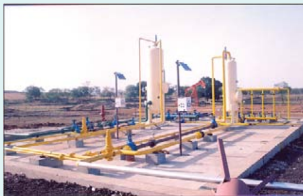
CBM Gas / Water Separation Facilities of RIL
